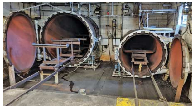
(2) 25' Gussett Vulcanizing Autoclaves
