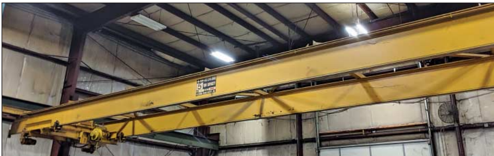
(3) 5 Ton x 55' Approx. Span PDS Underhung Overhead Bridge Cranes
