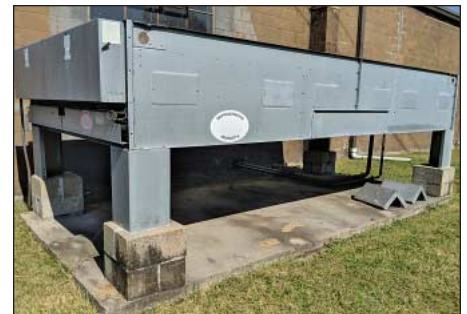
Thermal Care Model 8WMX Air Cooled Chiller
