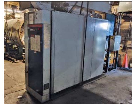
Miura Model LX-200 Steam Boiler
